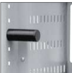
Tubular Cable Management Arms For Patch Cord Management
