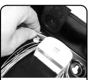
Terminate fiber according to manufacturer's specifications. Wrap fiber strands around the BRG2 as shown. Use lower section of BRG2 to store slack for adapter plates closest to floor of enclosure.
