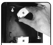
Install the Bend Radius Guide(BRG2)into position. Simply insert into square cut-outs and twist 45 degrees into locking position as shown.
